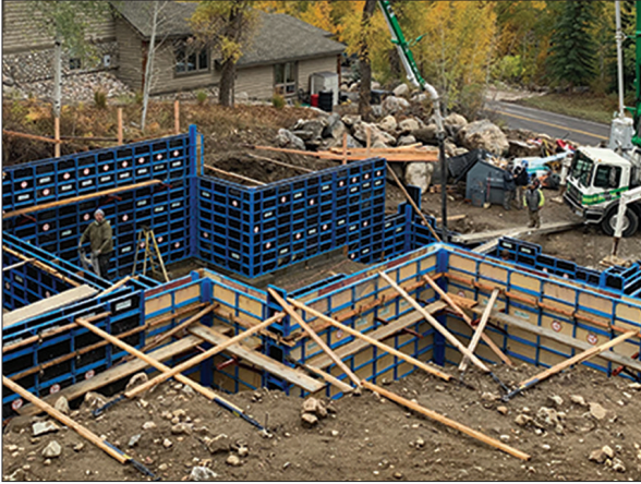
More dado slots along the side rail provide alternate tie locations “stepping” forms.
