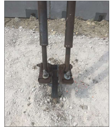
Pipe Braces attached to HGA Bracket for Double Brace Shoe on a Helical Ground Anchor
