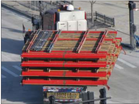
Gangforms are designed and preassembled before being delivered to the job site.
