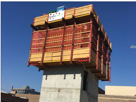
With the flip of a few switches, all interior and exterior formwork rises to the next level.
