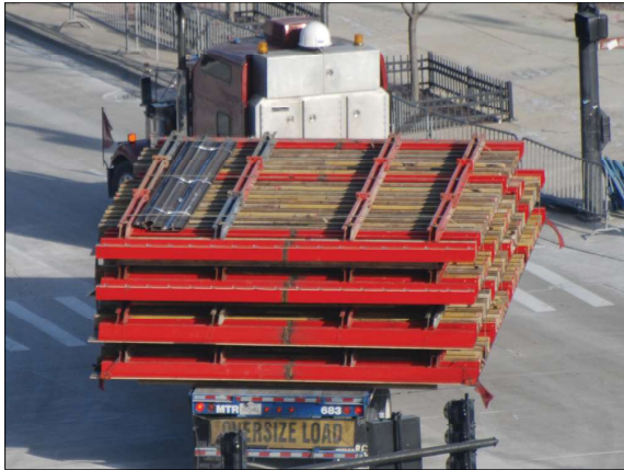
Gangforms are designed and preassembled before being delivered to the job site.
