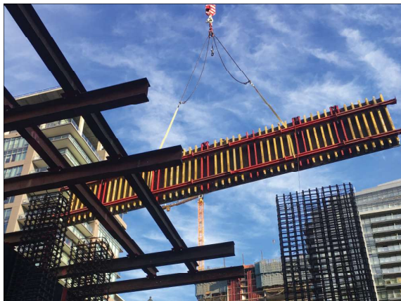
The forms are crane handled for the initial pour, but become part of the Self-Riser System for the remaining stories.
